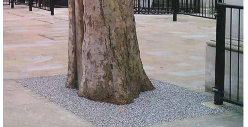
All of these gravels create an open texture that enables water to penetrate through the exterior surface, making it a fully porous system which is SuDS compliant.
